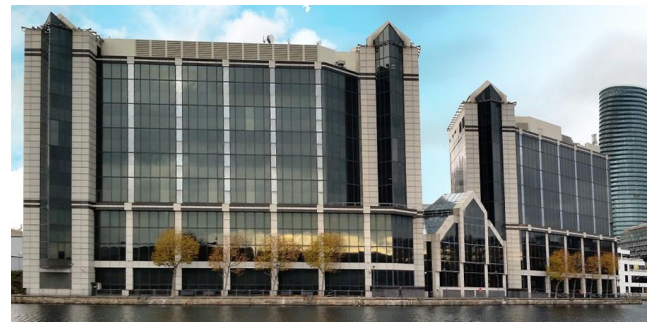
Telstra Security Centre (TSC) located at Telstra's London Hosting
